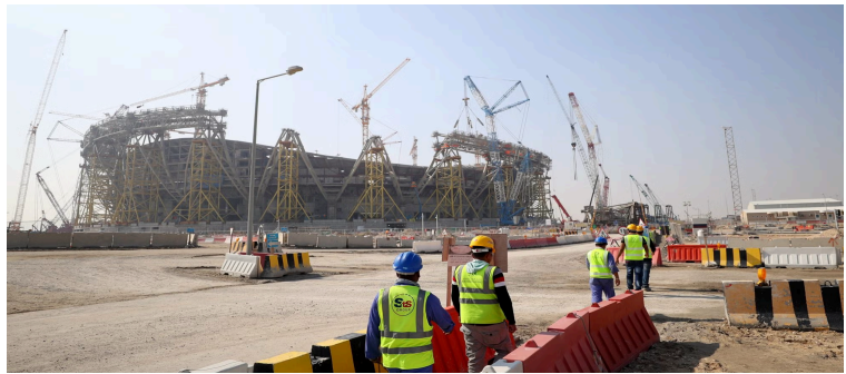
Figure 1: Construction workers at Qatar's World Cup Stadium Site (Georgetown Journal, 2023)
